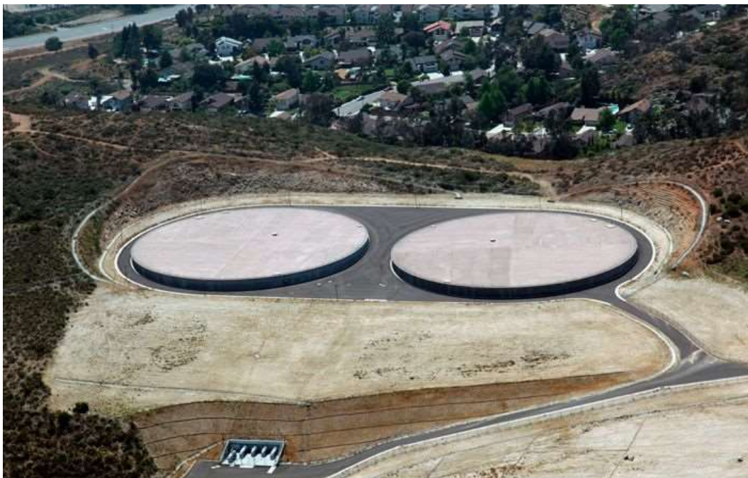
Figure 1.4 Aerial view of two concrete water storage tanks
