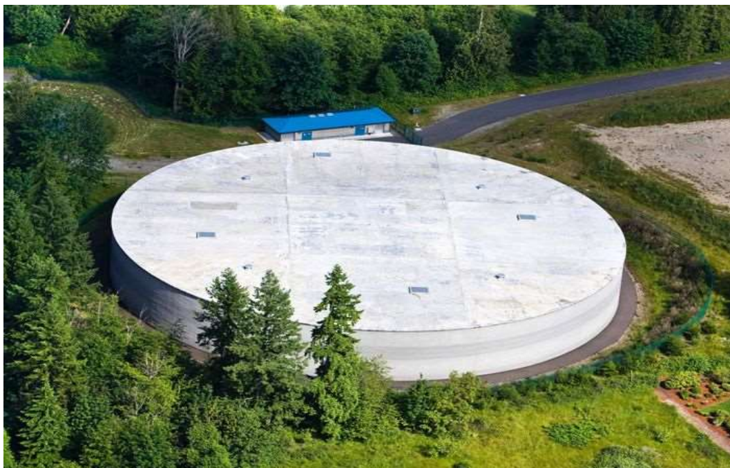
Figure 1.2 Concrete storage tank covered with a flat floor
