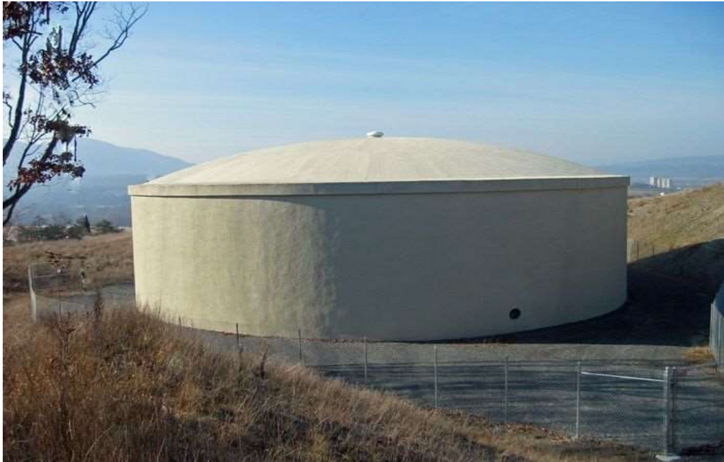
Figure 1.3 Concrete storage tank covered with a spherical dome
