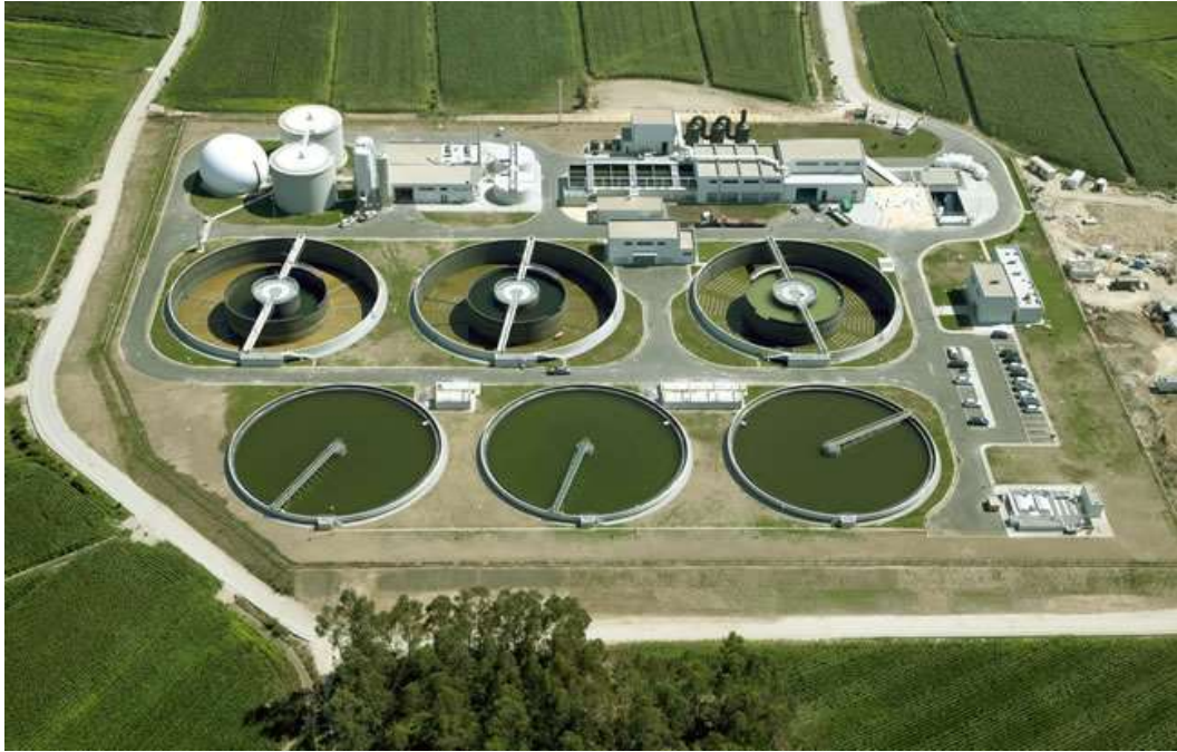
Figure 1.5 Aerial view of wastewater treatment plant
