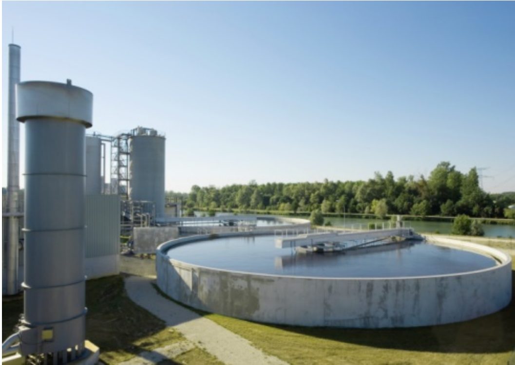
Figure 1.1 Opened concrete storage tank (Wastewater Treatment Plant)
